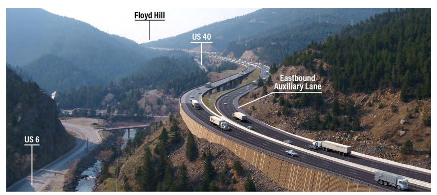
At the Beaver Brook/Floyd Hill and Hyland Hills/Floyd Hill interchange system, the split-diamond interchange configuration (with on- and off-ramps connected by US 40) would remain, and no new accesses would be provided. However, the US 40 Roundabouts project, planned
