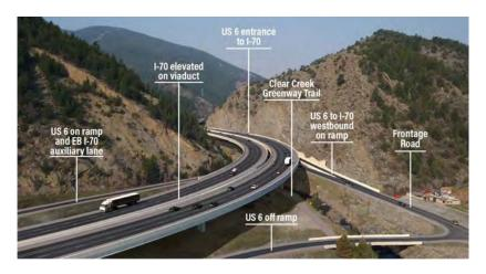
As illustrated in <u>Exhibit 3-8</u>, realigning the roadway on the south side of the canyon would avoid existing tight curves around the two hills between the US 6 interchange and the Hidden Valley/Central City interchange (west of the view in <u>Exhibit 3-6</u>). Elevating I-70 would provide more space in the canyon for the new frontage road (allowing it to be constructed generally within the existing I-70 pavement), creek, and wildlife movement and would create opportunities for
